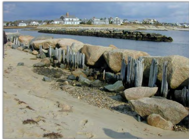
Photograph 2.1. Coastal beach with jetty. Although there is a jetty on this beach, the sand is still able to respond to wave/water activity by shifting and changing form as seen from the sand that is being eroded from behind the jetty. The amount of sediment exchange between the beach on the left and right of the rocks, however, has been restricted by the jetty.
