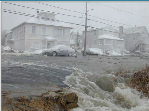
Photograph 2.20. Land subject to coastal storm flowage with diminished ability to slow flood waters or reduce storm-wave overwash. The solid foundations and pavement in this area of land subject to coastal storm flowage has led to an increased velocity of storm-wave overwash and a channeling of flood waters toward landward areas. 72 In this picture, the ocean is behind the houses (that are on a developed and altered dune). In such an area where the dune has lost most of its ability to exchange sediment with the beach and dissipate wave energy, it is all the more important to protect the functions of land subject to coastal storm flowage. Photograph courtesy of Margo Clerkin, former Hull Conservation Agent.
