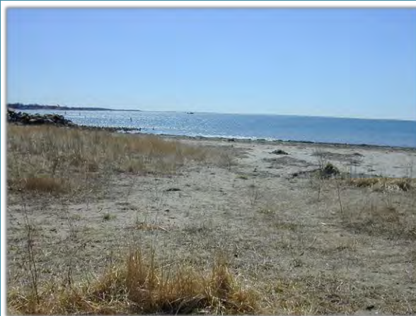
Photograph 2.13. Low volume dune. Relative to the beach, this is a mound or ridge of sand deposited by wind and/or waves. This dune provides an area for dissipation of storm wave energy, but will not provide enough volume to prevent high energy waves from extending farther landward. The dune still has the ability to erode and shift and move landward and laterally.
