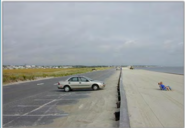
Photograph 2.9. Modified dune form. This parking lot and seawall have significantly modified the dune form and have diminished its capacity to shift and change form to dissipate wave energy. In storm events, the flood water and waves will increase in velocity as they move across the pavement and likely extend farther landward than if no pavement was present. The vegetated dune landward of the parking lot can still dissipate wave energy through the friction of the vegetation and by shifting and changing form in a storm event.
