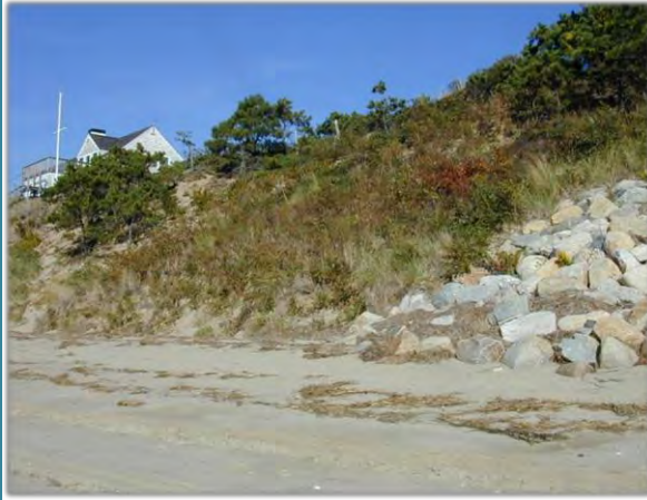
Photograph 2.16. Coastal bank (with riprap) serving as a sediment source and a vertical buffer. In spite of the riprap, this coastal bank does act as a sediment source to the adjacent beach, since wave activity can erode the bank. The bank can also function as a vertical buffer due to its height, and can withstand erosion from wind and rain because of the stabilizing vegetation.
