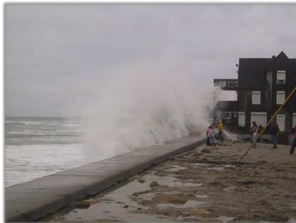
Photograph 2.22. Land subject to coastal storm flowage with diminished ability to reduce wave energy. Here, a coastal engineering structure deflects, reflects, and redirects storm waves, affecting adjacent properties, landward areas, and the subject property with wave energy, overwash, and flood waters. The pavement in this area of land subject to coastal storm flowage has also led to an increased velocity of storm-wave overwash and a channeling of flood waters toward landward areas.
